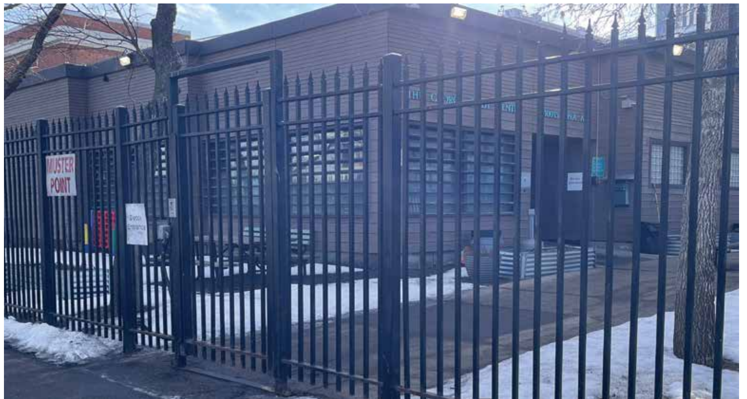
The George Spady Centre in its current location at 10015 105A Avenue. Paula E. Kirman
